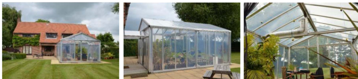
Fig. 4. The external and internal views of a structure with ETFE encapsulated panels: external skin built at the garden of a detached house used as an outdoor room and a greenhouse for plants. (Source: Masih et al. [66]).
